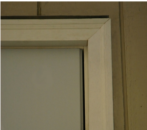
Figure 29. Shows standard “Brickmold” casing at existing door unit with siding.
