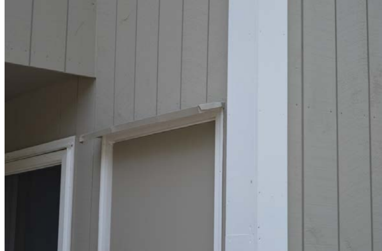
Figure 34. Rain Shield over exterior closet
