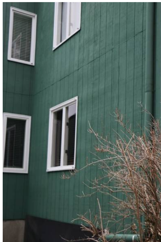
Figure 30. Wall re-sided with T1-11
