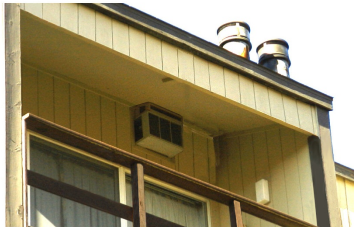
Figure 1 AC unit over sliding door
