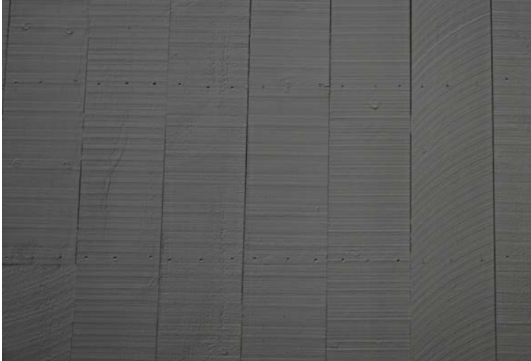
Figure 27. Style 1 siding, rough sawn lumber with little groove between boards
