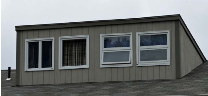
Figure 26. Examples of the three types of acceptable clearstory windows, Casement on the left, Single pane either fixed or awning, and double awning windows. In all cases the windows must match the original windows in size. Trim details and spacing needs to be maintained, i.e. no window units mulled together with only trim between windows
