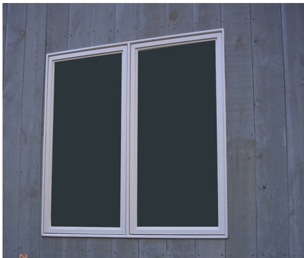
Figure 24. New vinyl casement window installed without trim.
