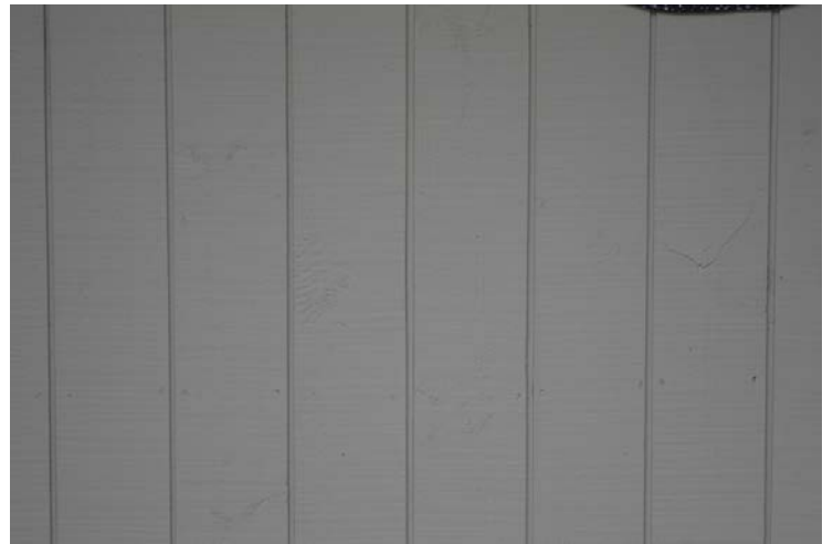
Figure 28. Style 2 siding, rough sawn lumber with wider groove between boards
