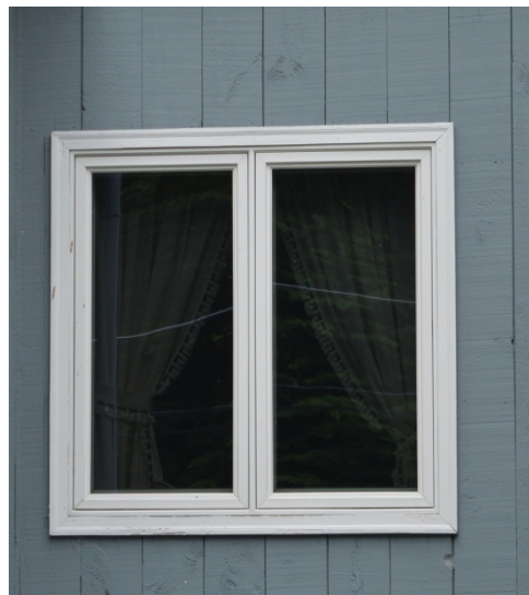
Figure 25. New vinyl casement window trimmed in brickmold.
