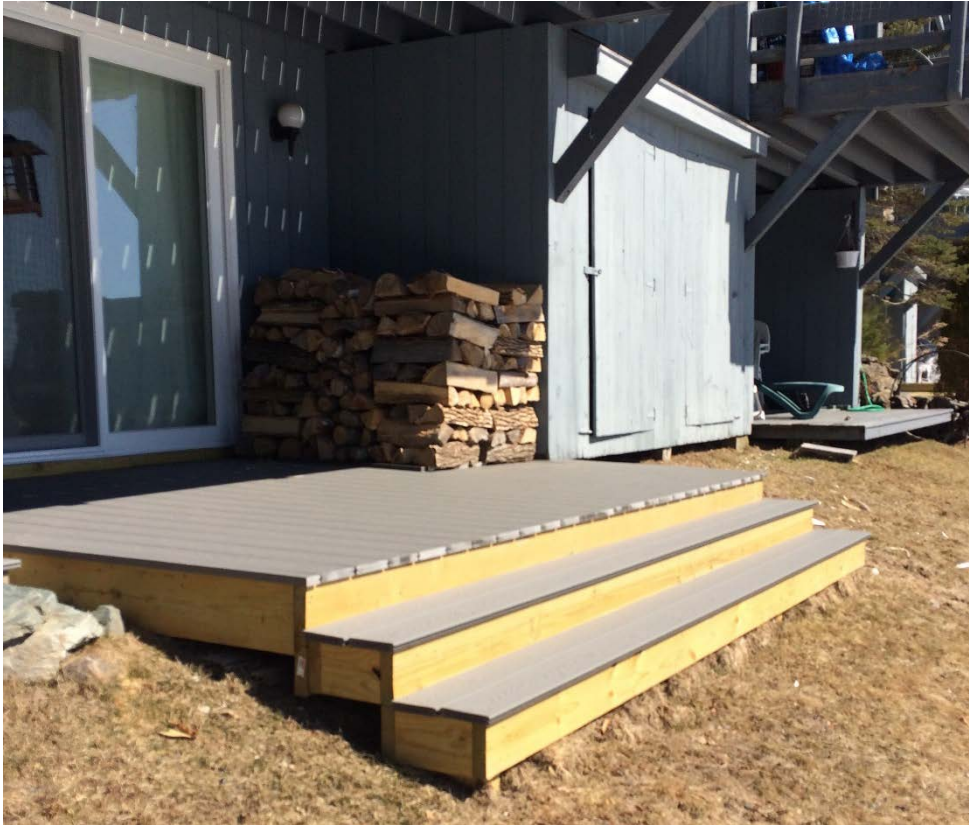
Figure 12. Photo shows basement level decks on type B buildings. Deck in background shows deck with no step and deck in foreground shows deck with steps required because of slope of land
