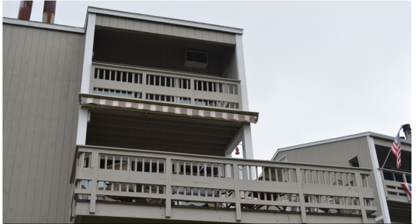
Figure 11. Original top, bottom and intermediate rails with balusters applied to inside face
