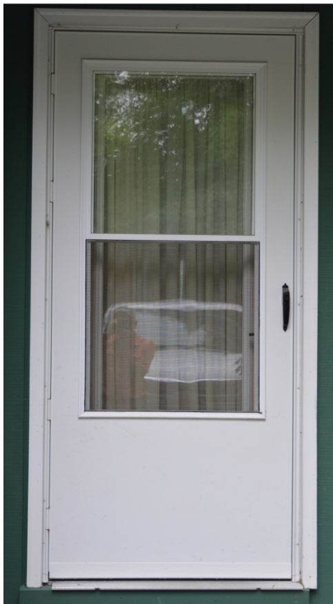
Figure 21. 2/3 Light storm door
