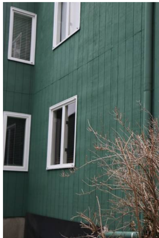
Figure 29. Wall re-sided with T1-11
