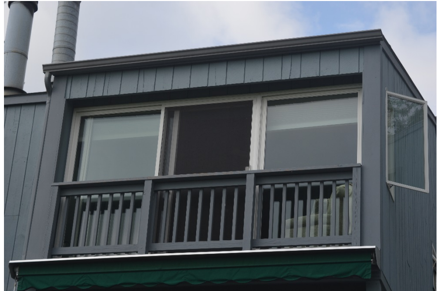
Figure 15. Type B 2 nd Floor Deck Enclosure
