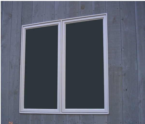
Figure 23. New vinyl casement window installed without trim.
