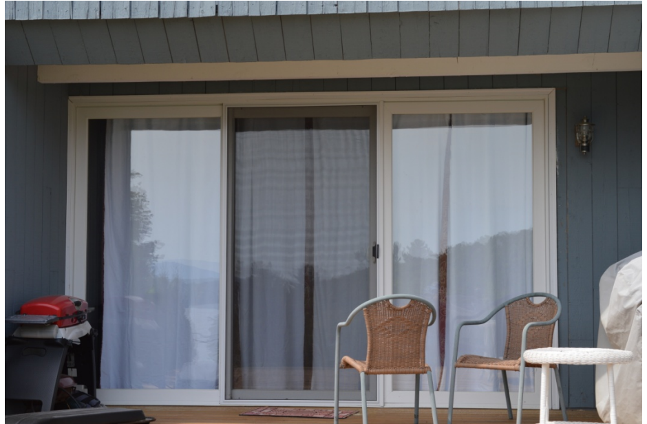
Figure 16. Typical 3 panel 8' high by 12' wide
