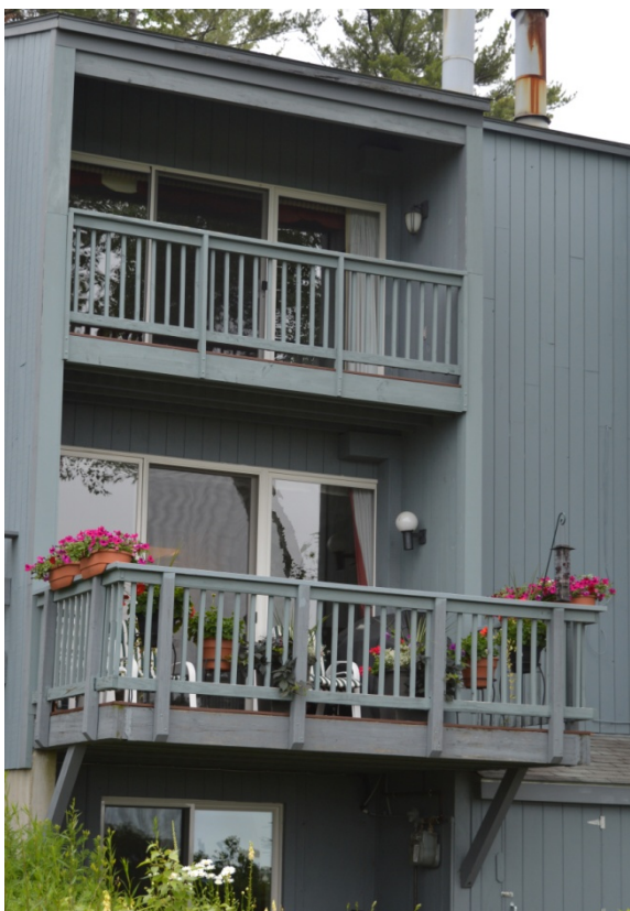
Figure 10. Top and bottom rails with balusters
