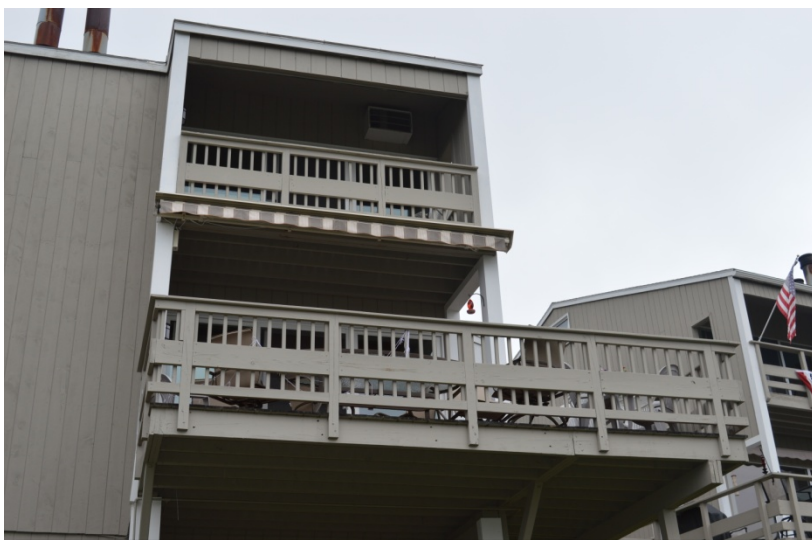
Figure 11. Original top, bottom and intermediate rails with balusters applied to inside face
