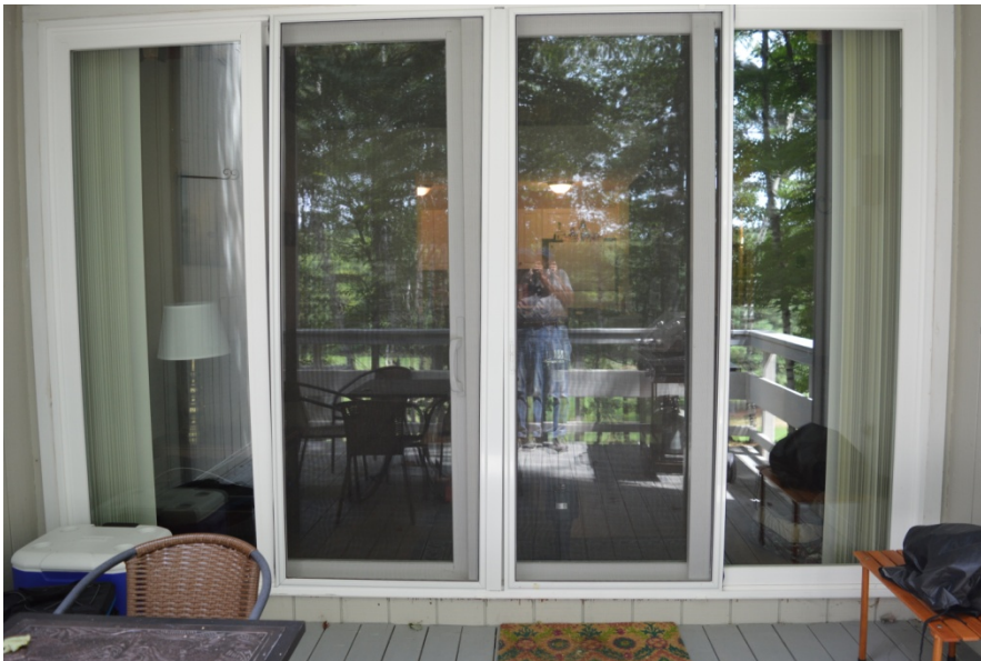
Figure 17. Acceptable 4 panel 8' high by 12' wide sliding door
