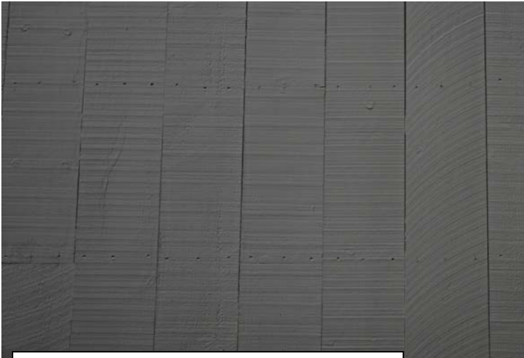
Figure 26. Style 1 siding, rough sawn lumber with little groove between boards.
