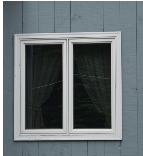
Figure 24. New vinyl casement window trimmed in brickmold.
