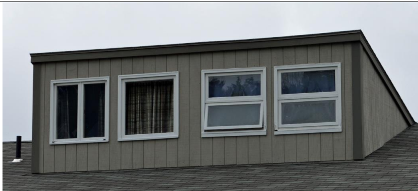
Figure 23. Examples of the three types of acceptable clearstory windows, Casement on the left, Single pane either fixed or awning, and double awning windows. In all cases the windows must match the original windows in size. Trim details and spacing needs to be maintained, ie no window units mulled together with only trim between windows
