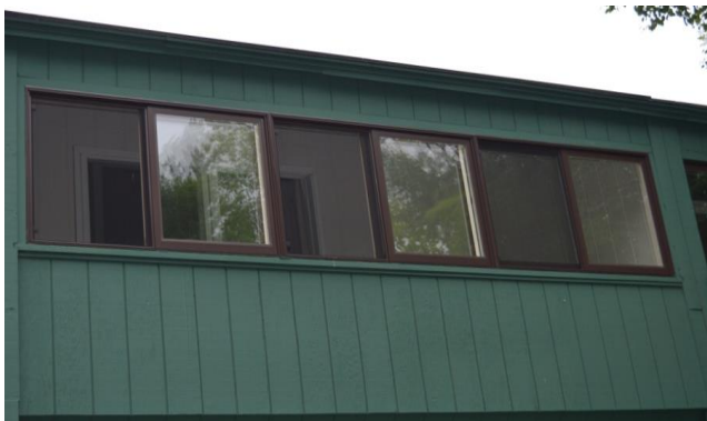
Figure 12. Type A unit 2 nd Floor deck Enclosure
