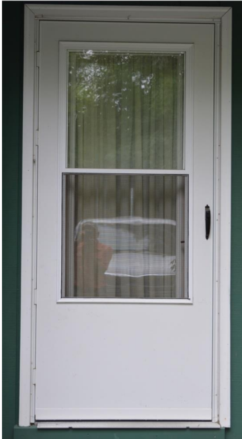
Figure 19 . 2/3 Light storm door
