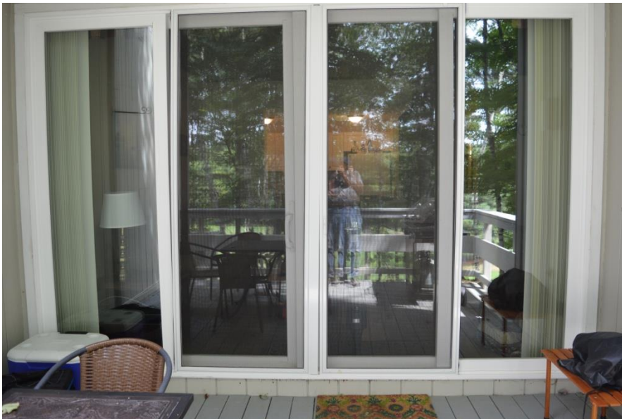
Figure 15. Acceptable 4 panel 8' high by 12' wide sliding door
