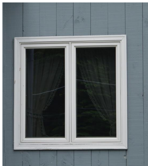
Figure 22. New vinyl casement window trimmed in brickmold.
