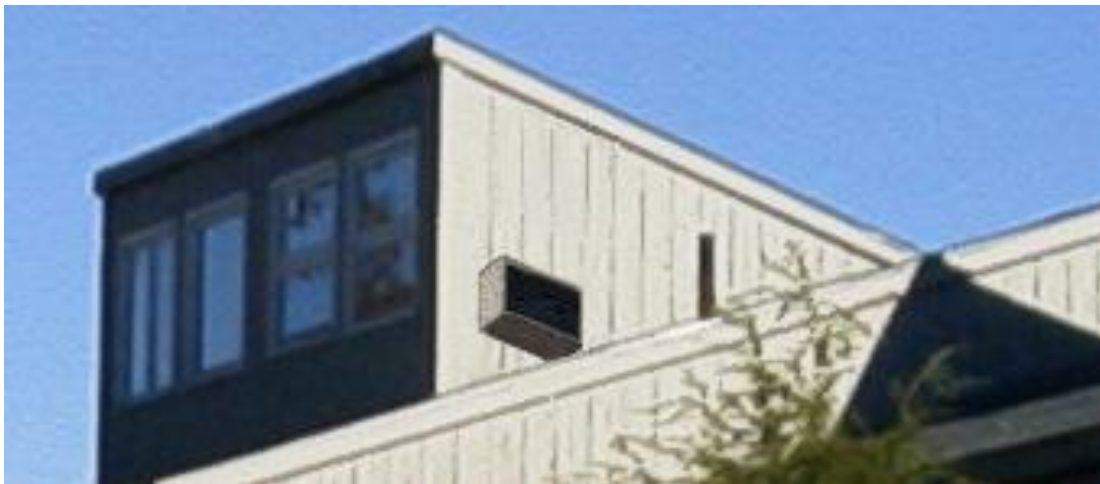
Figure 3. location of AC unit in dormer sidewall of Type 'B' unit.
