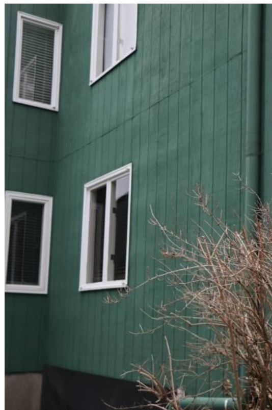
Figure 27. Wall re-sided with T1-11
