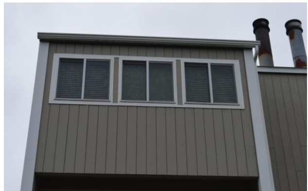
Figure 13. Type B unit 2 nd Floor deck Enclosure
