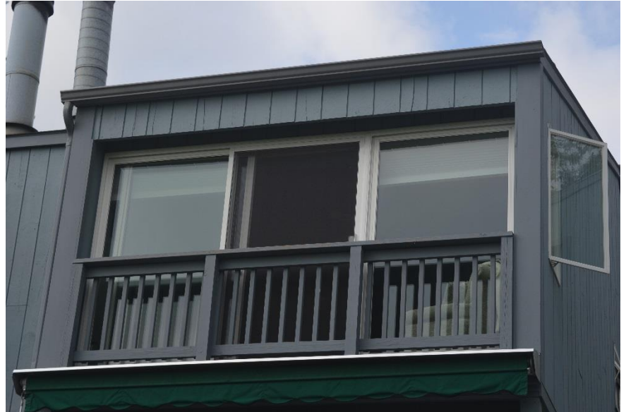
Figure 16. Type B 2 nd Floor Deck Enclosure
